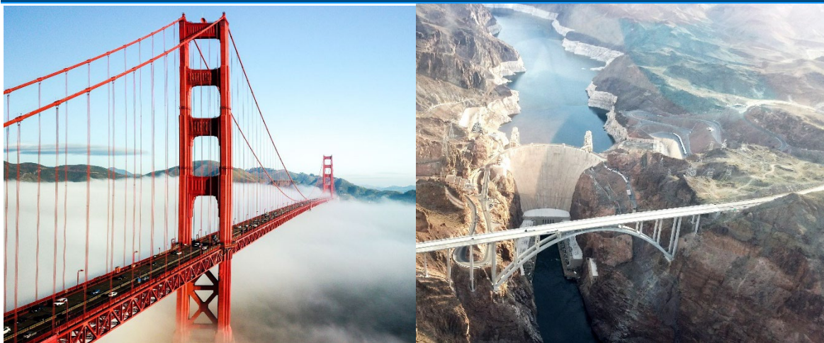
Figure 11 Suspension and arch bridges
