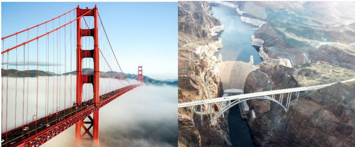
Figure 11 Suspension and arch bridges
